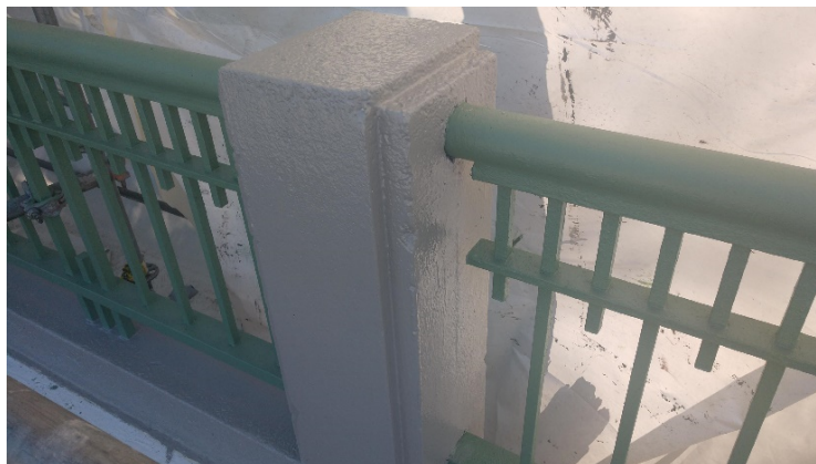
Main Street Bridge - Painted Railings and Pillars
