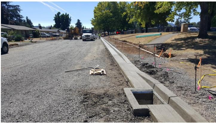
The concrete crew will be on site for two days next week. They will focusing on "tie-ins". This is the space between the existing curb and gutter and the new curb in gutter. This work will be hand formed and pour.
