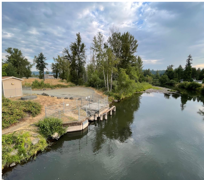
Row River intake
