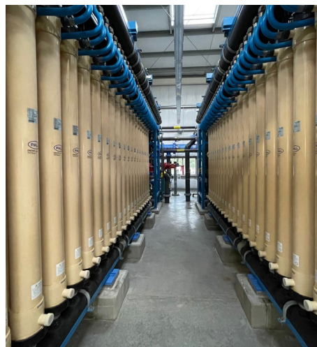
Left: The 2022 water treatment plant staff. Middle: The three filtration racks at the water treatment plant have a production capacity of 6 million gallons per day. Having three filtration racks makes maintenance on the filtration system more efficient and keeps our produced drinking water at the highest quality possible. Right: New bulk water storage tanks.
