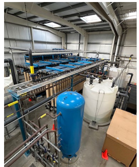
Left: The 2023 water treatment plant staff. Middle: The three filtration racks at the water treatment plant have a production capacity of 6 million gallons per day. Having three filtration racks makes maintenance on the filtration system more efficient and keeps our produced drinking water at the highest quality possible. Right: The bulk water storage tanks.
