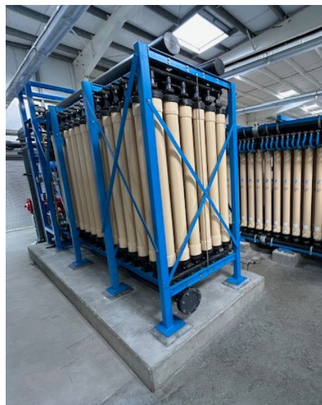
Left: The 2023 water treatment plant staff. Middle: The three filtration racks at the water treatment plant have a production capacity of 6 million gallons per day. Having three filtration racks makes maintenance on the filtration system more efficient and keeps our produced drinking water at the highest quality possible. Right: The bulk water storage tanks.
