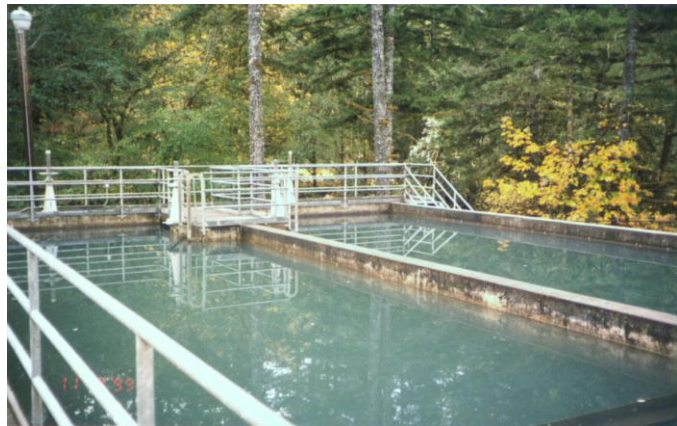
View of inlet end of settling tanks
