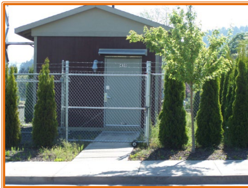
Telecom Hut located on South 6 th Street
