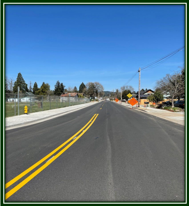
Completed South 4 th Street Safe Sidewalk project
