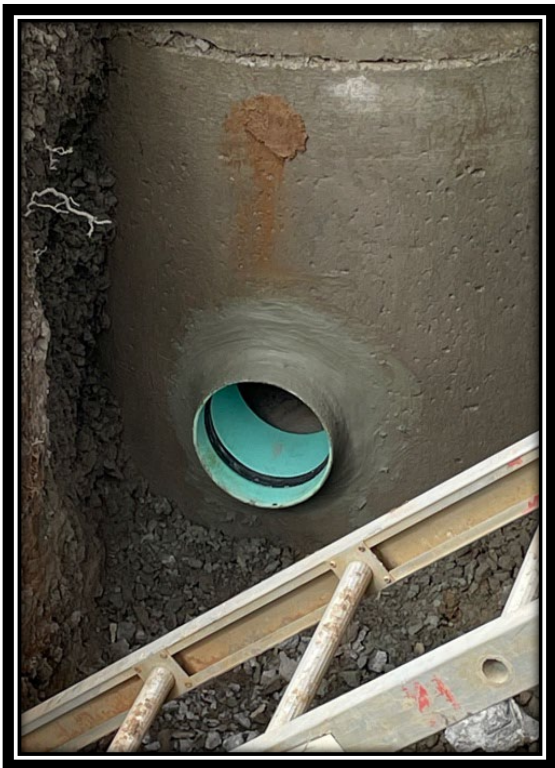
New sewer mainline installation on S. 12 th Street
