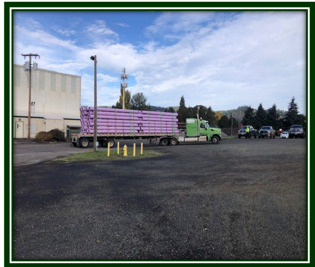
2,000' of 12" Effluent Pipe for Line to Trailhead Park
