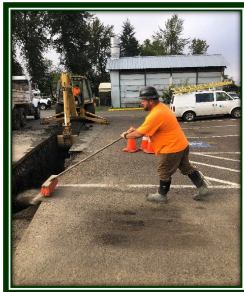
City crew replacing storm drainage line at City Shop
