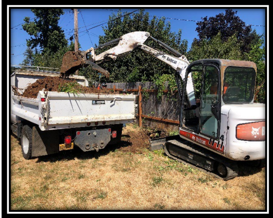
Back lot sewer lateral failure repair at 241 M Street
