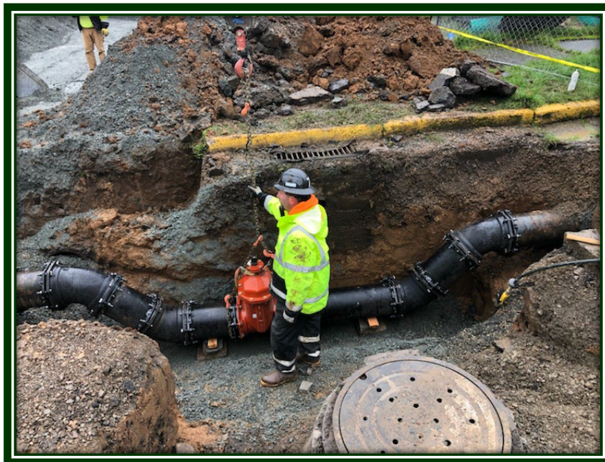
Utility crew moving water mainline for Harrison Apartments project
