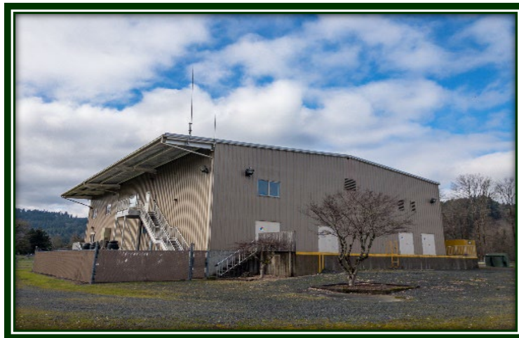
An exterior view of the Row River Water Treatment Plant
