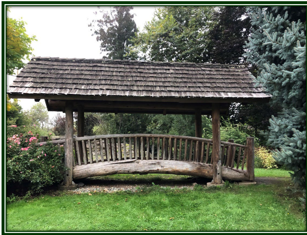
Donated Covered Bridge from the Village Green to be installed at the golf course
